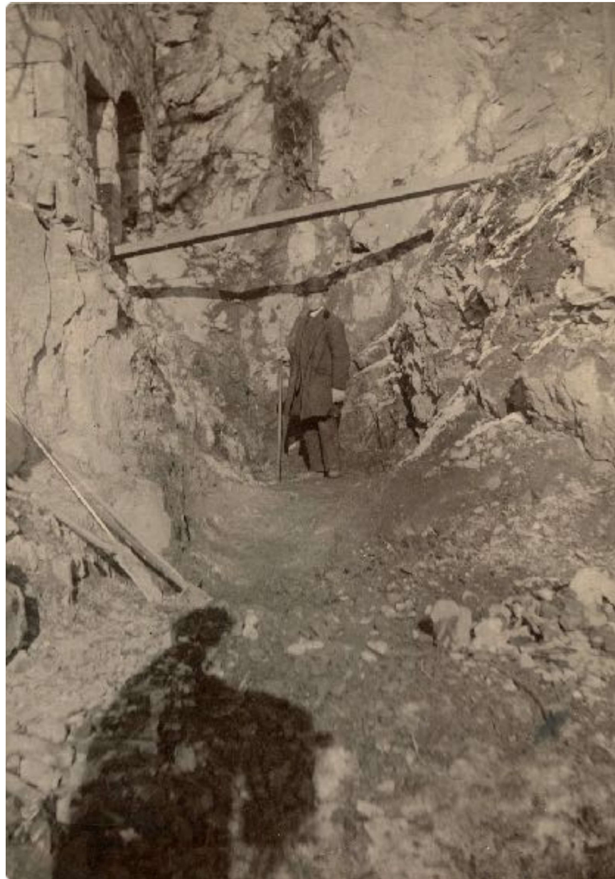
L.F. Benton in flume prior to construction.
